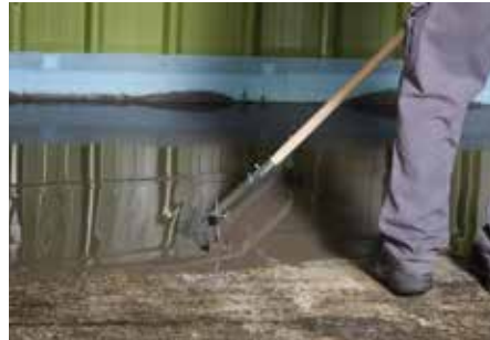
5 While working larger areas use a KÖSTER Gauging Rake to distribute the material
