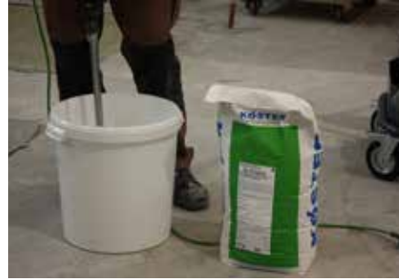
3 Use an electrical paddle mixer and mix intensively for three minutes
